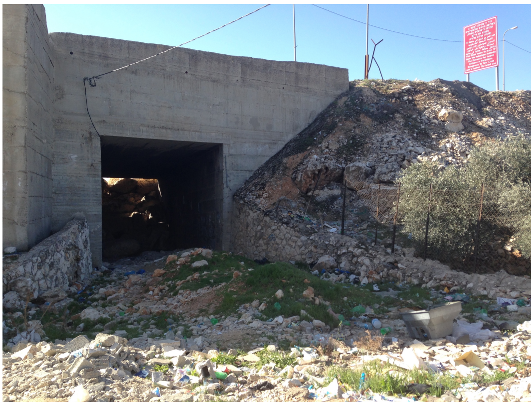
Figure 2.4 Blocked tunnel to the entrance of Jaba' Source: Callie Maidhof, Feb. 28, 2014 28
